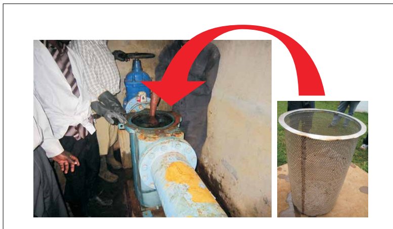
Photo 4.1 installation of Strainer
