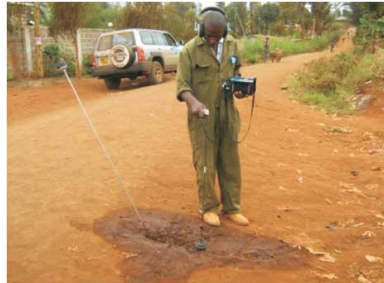
Photo 2.14: Leak detection using Electronic leak detector
