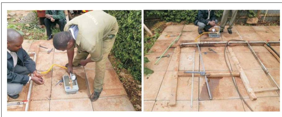
Photo 2.27: Water pressure test on service line model
