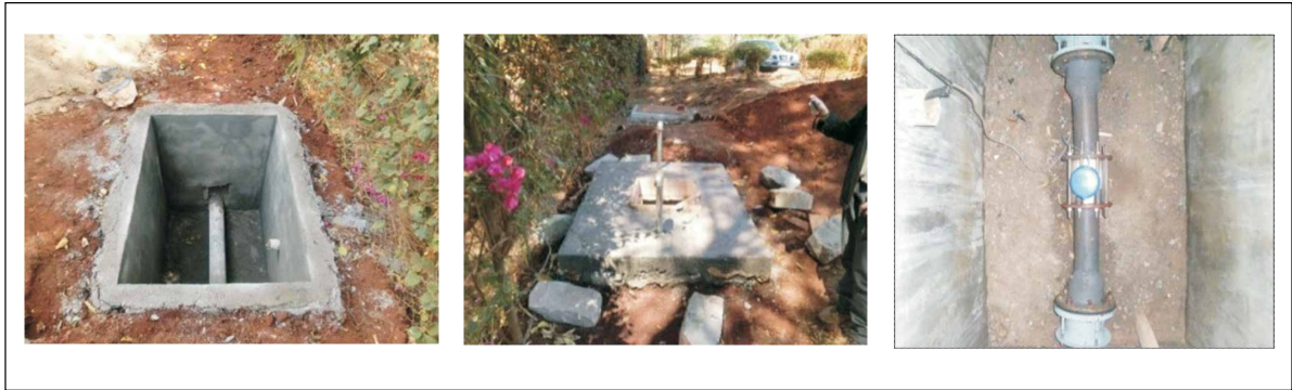
Photo 2.1 Construction and install of New Master meter and chamber
