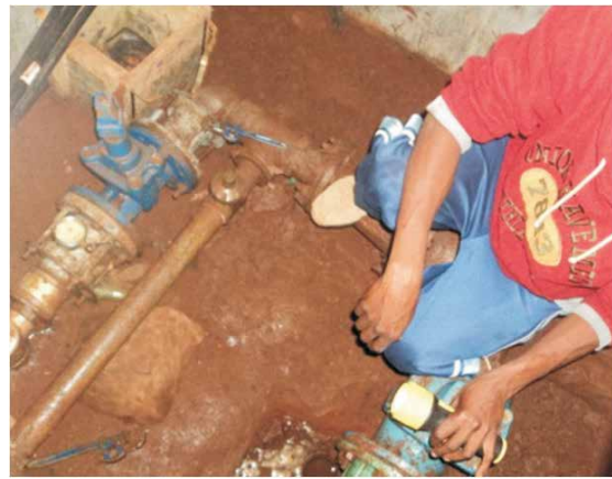
Photo 2.7: Measure the flow rate into the block
