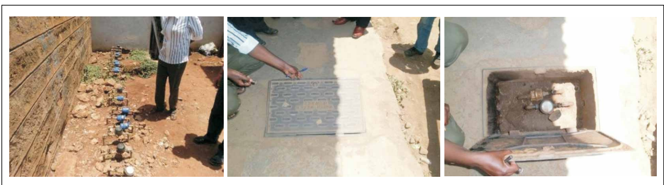
Photo 5.6 Placement of the meter
