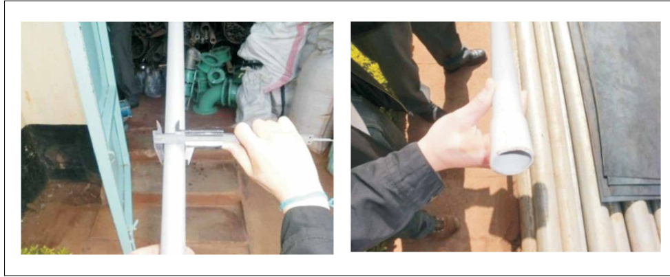
Photo 2.24: Measuring pipe diameter
