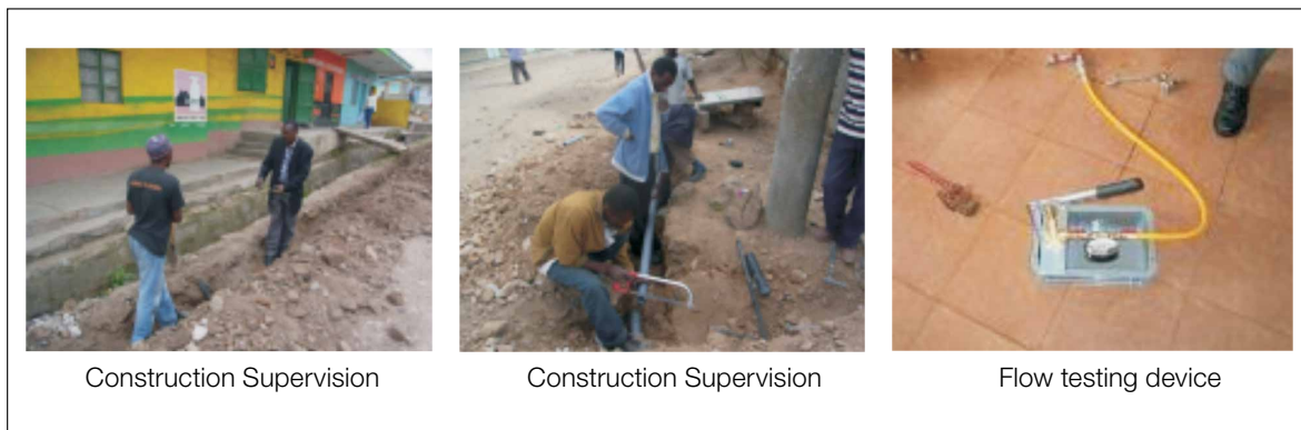
Photo 3.2 Construction supervision and flow testing device
