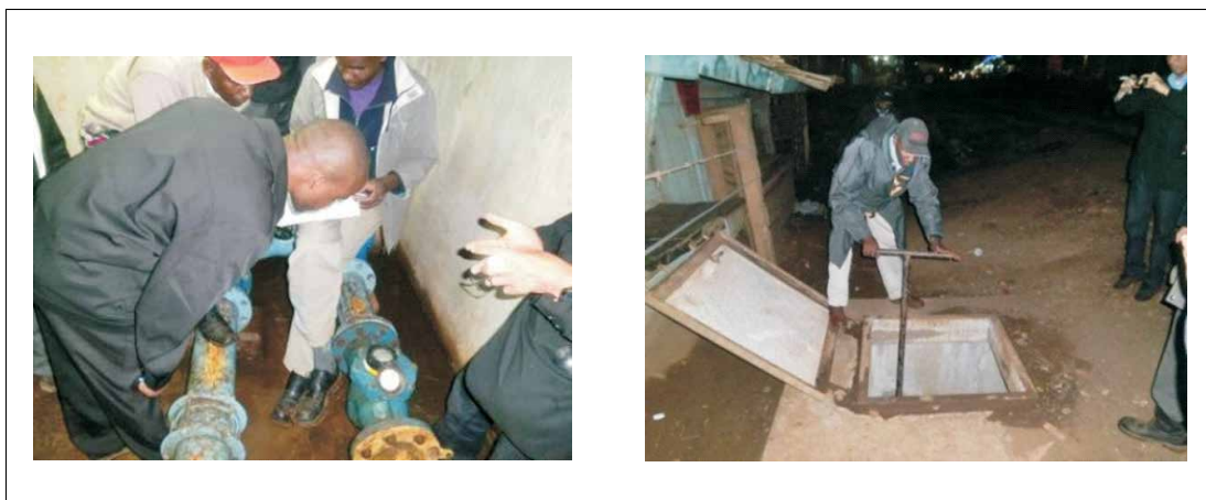
Photo 5.2 Step test measurement (Left: measuring flow volume, Right: Closing gate valve)
