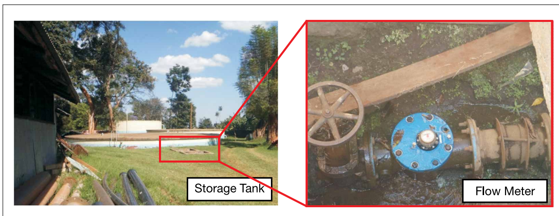
Photo 1.1: Installation of Flow Meter at Outlet of Storage Tanks
