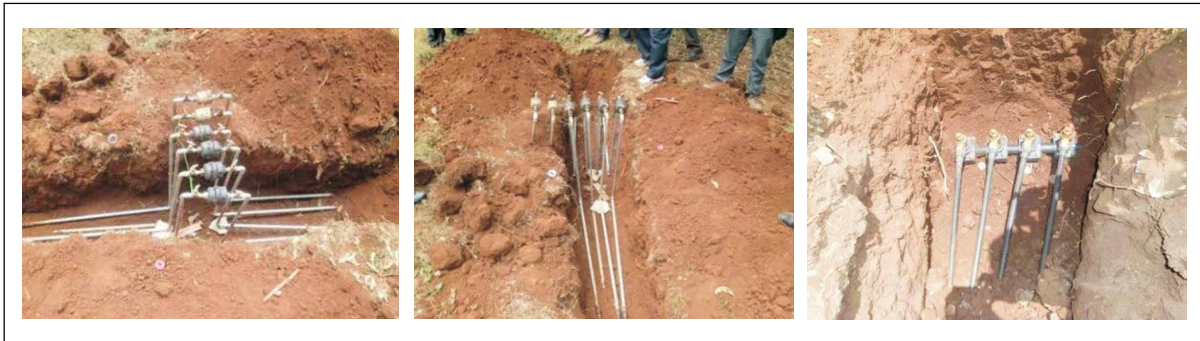
Photo 5.7 Placement of Service Pipe
