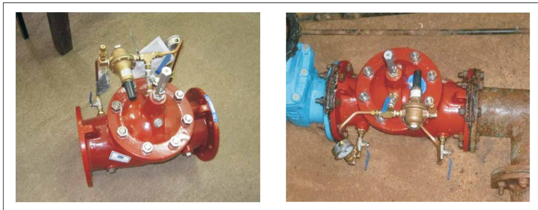
Photo 2.22: Installation of Auto PRV (large type)
