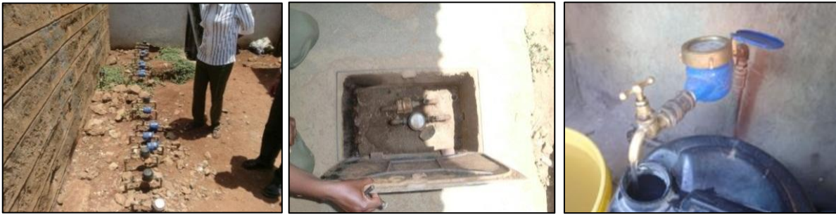
Figure 6.10: Actual Installation of Customer Water Meter
