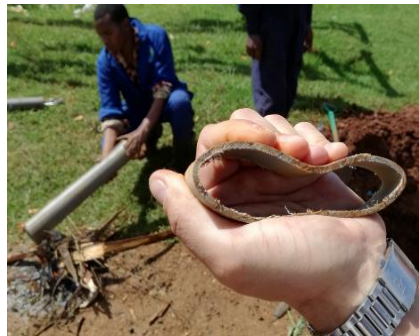
Figure 8.9: Degradation of pipe caused by excessive heat on the UPVC pipe.
