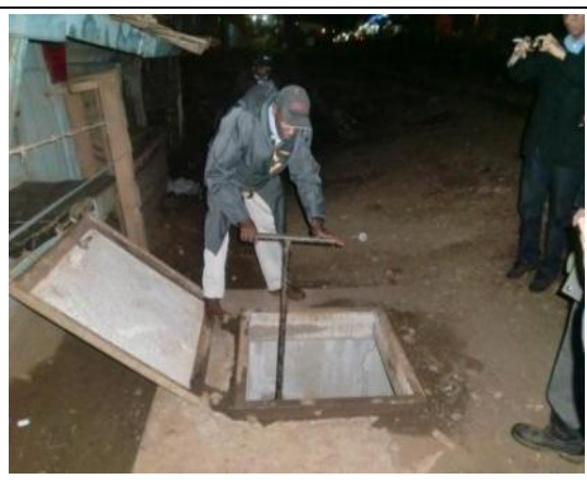
Figure 9.9: Closing Gate Valve
