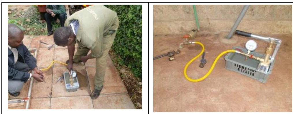
Figure 8.17 Water Pressure Test
