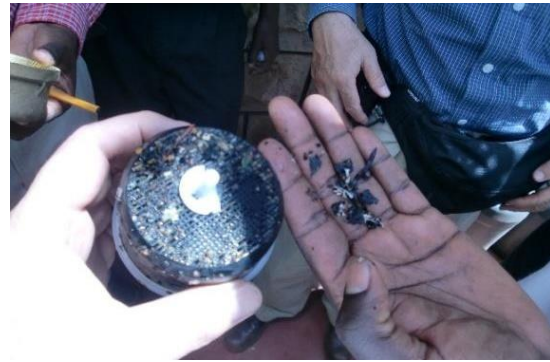
Figure 6.2: Roots at Customer Meter (Embu WSP)
