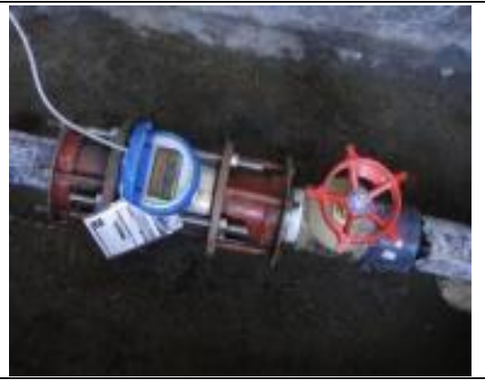
Figure 8.6: Measure the flow volume into the block
