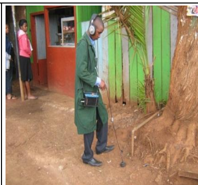
Figure 9.19: Leak detection using electronic leak detector
