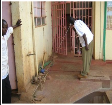
Figure 9.15: Leak detection using Listening Stick
