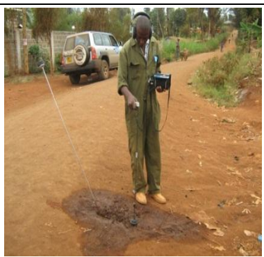
Figure 9.18: Leak detection using electronic leak detector
