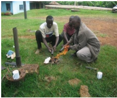
Figure 8.8: Making Fire Coupling (used for pipe connections in Kenya)
