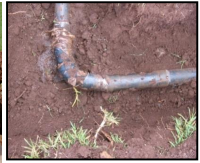
Figure 8.10: Plastic Pipe Bend (used for pipe connections in Kenya)
