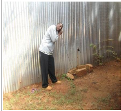
Figure 9.16: Leak detection using Listening Stick
