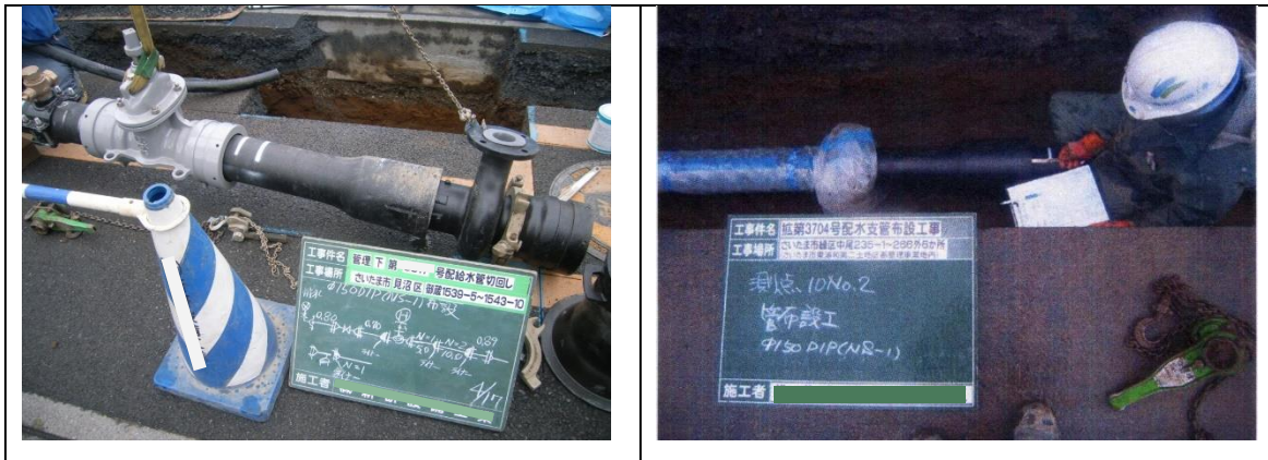
Figure 8.16: Connection work of Pipe (Japanese Case)
