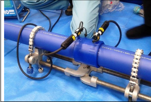
Fig. 2.25: Electrofusion Welding in progress
