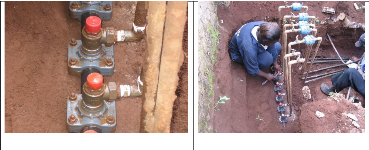
Fig. 3.1: Tapping with standardized saddle clamp and ferrule (tap)
