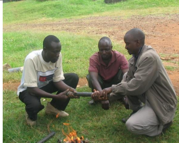
Fig. 2.14: Making Fire Coupling from Softened Pipes
