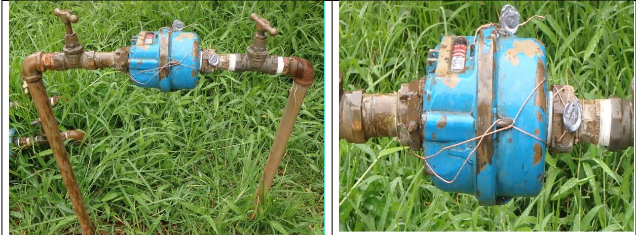
Fig. 8.8: Meter sealed by sealing wire and sealing lead
