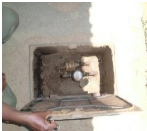
Photo 3.2: Installation of Customer Meters in a meter box
