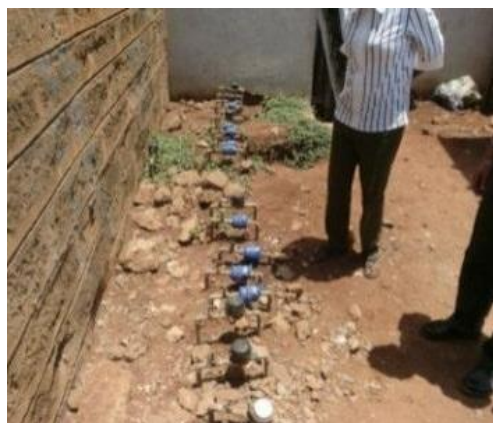
Photo 3.1: Installation of Customer Meters without meter box
