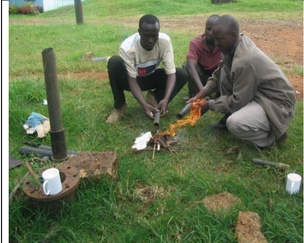
Fig. 2.13: Softening Pipe by Heating
