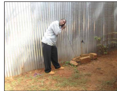
Photo 3.10: Leak detection using Listening Stick
