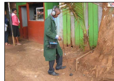
Photo 3.13: Leak detection using electronic leak detector
