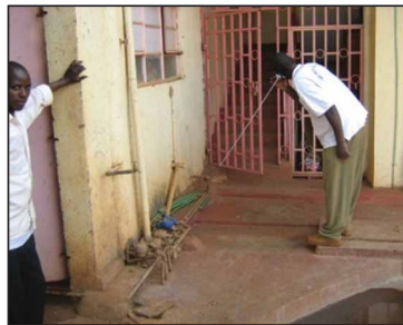
Photo 3.9: Leak detection using Listening Stick
