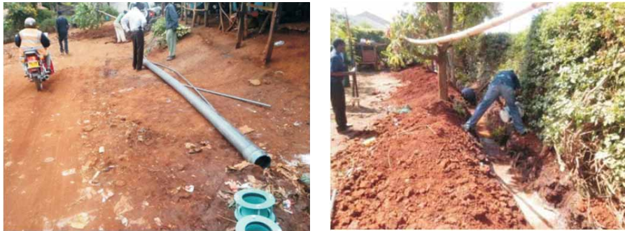
Photo 5.14: Replacement of Distribution Pipes
