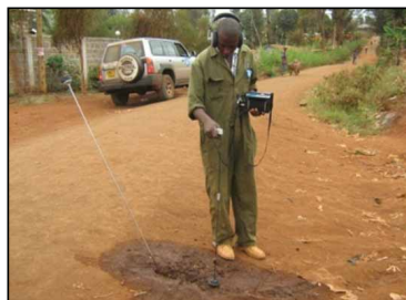
Photo 3.12: Leak detection using electronic leak detector
