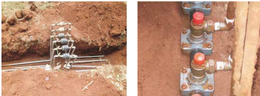
Photo 5.15: Replacement of Service Pipes
