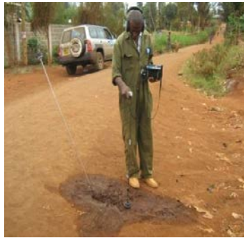
Figure 9.18: Leak detection using electronic leak detector
