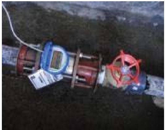
Figure 8.6: Measure the flow volume into the block
