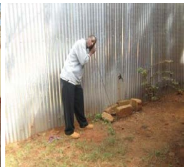
Figure 9.16: Leak detection using Listening Stick
