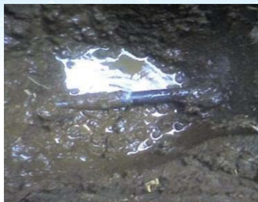
Figure 8.3: Underground (Invisible) Leakage
