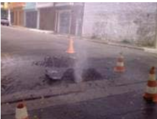
Figure 8.2: Visible Leakage (Surface leakage)
