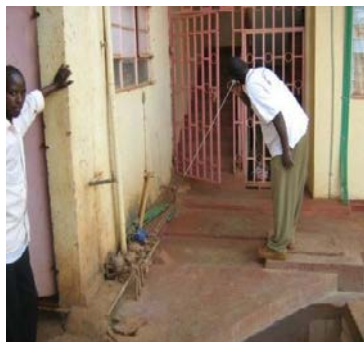
Figure 9.15: Leak detection using Listening Stick
