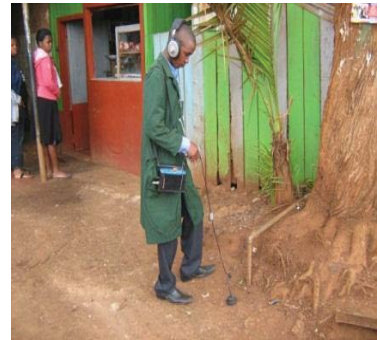
Figure 9.19: Leak detection using electronic leak detector
