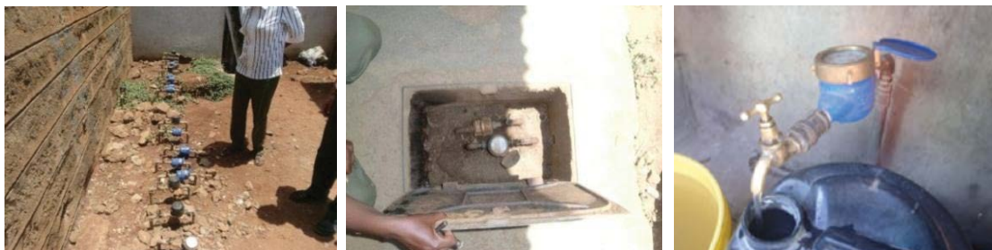
Figure 6.10: Actual Installation of Customer Water Meter
