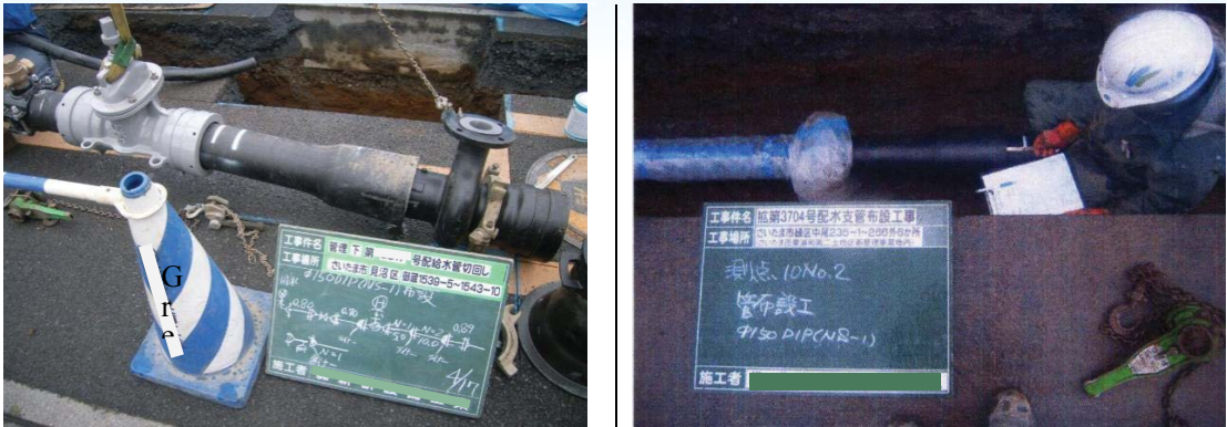
Figure 8.16: Connection work of Pipe (Japanese Case)
