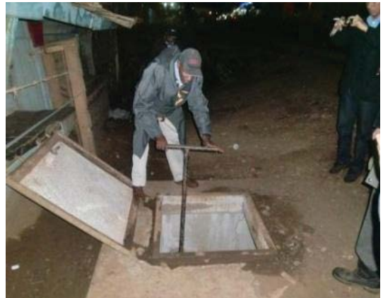
Figure 9.9: Closing Gate Valve
